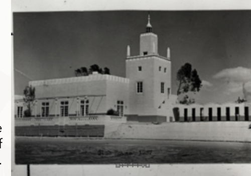
An early view of the Clubhouse with a row of changing rooms to the side.
