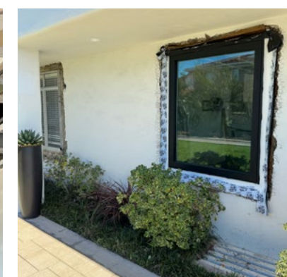
Modern black metal windows replace the 25 year-old leaky aluminum windows
