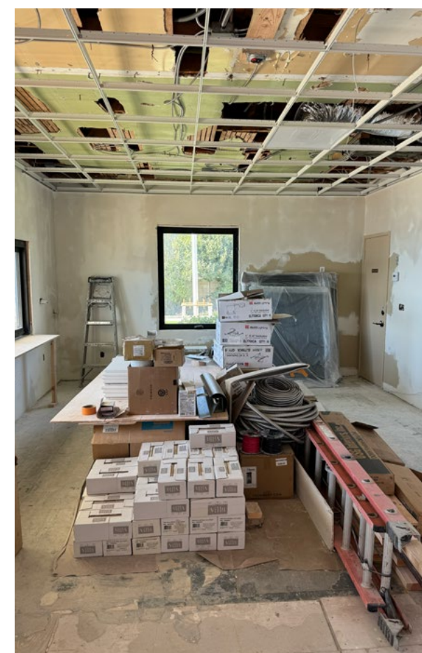
The Board Room Under Construction
