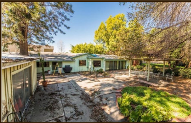
A modern view of Ellerbroek's traditional 1952 home on Dodge Ave., Tustin.
