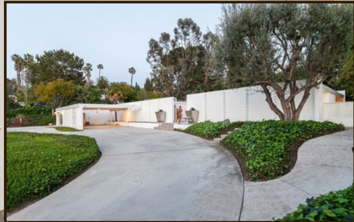
Ellerbroek's Cielo Place residence in North Tustin dating from 1961.
