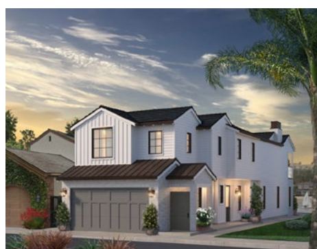
VIA LIDO NORD - LIDO ISLE Under Construction - Private Residence
