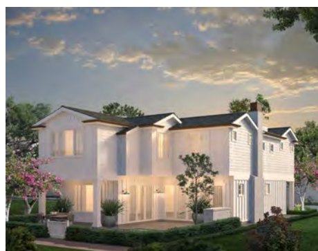
VIA ITHACA - LIDO ISLE Under Construction - Available
