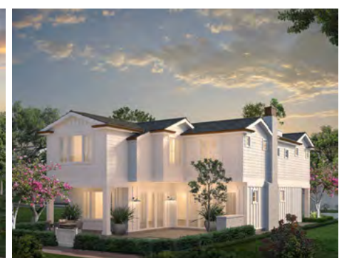
VIA ITHACA - LIDO ISLE Under Construction - Available
